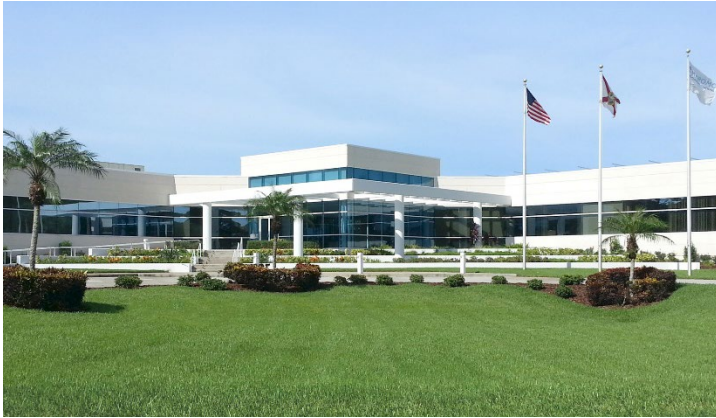
FAULHABER MICROMO LLC located in Clearwater, FL USA fmo_building.jpg © FAULHABER
